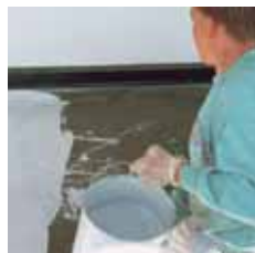
StoPur EB 200 felhordása
