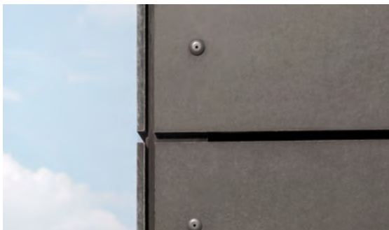
Visible mounting of the fibre cement panels with coloured rivets
