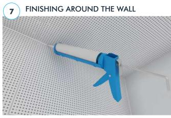
Finish the surface using silicone sealant around the perimeter.
